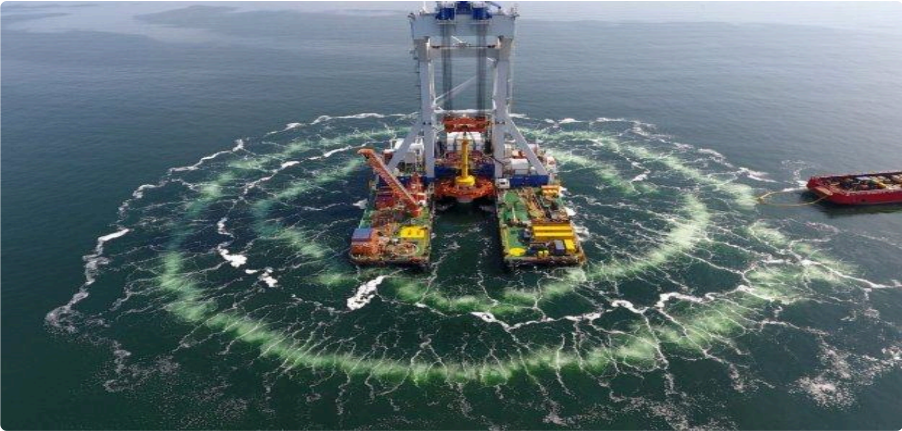
Big Bubble Curtain deployed on pile driving for Vineyard Wind 1
